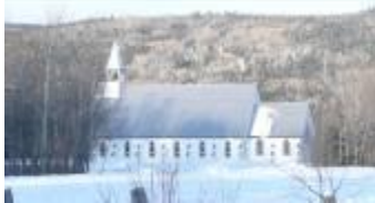
Figure 5.48 St.Andrew's Anglican Church
