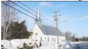
Figure 5.41 St.James Anglican Church
